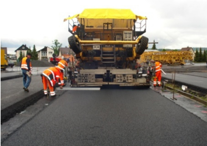
Figure 10: Surface of wearing course on testing ground 3 (mod. compact asphalt 22+2 cm) before roller compaction
