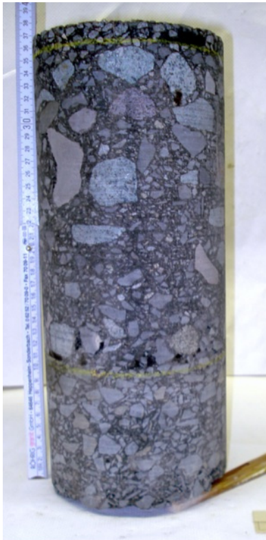
Figure 13: Core from testing ground 3 (mod. compact asphalt 22+2 cm on asphalt base)
