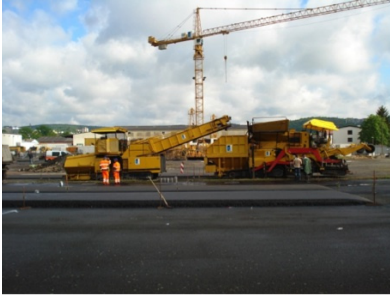
Figure 8: Paving on testing grounds
