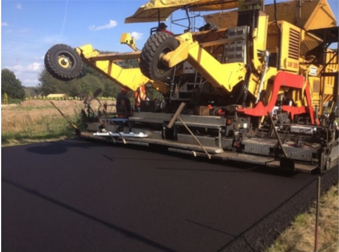
Figure 19: Paving of modified compact asphalt on test track B 68
